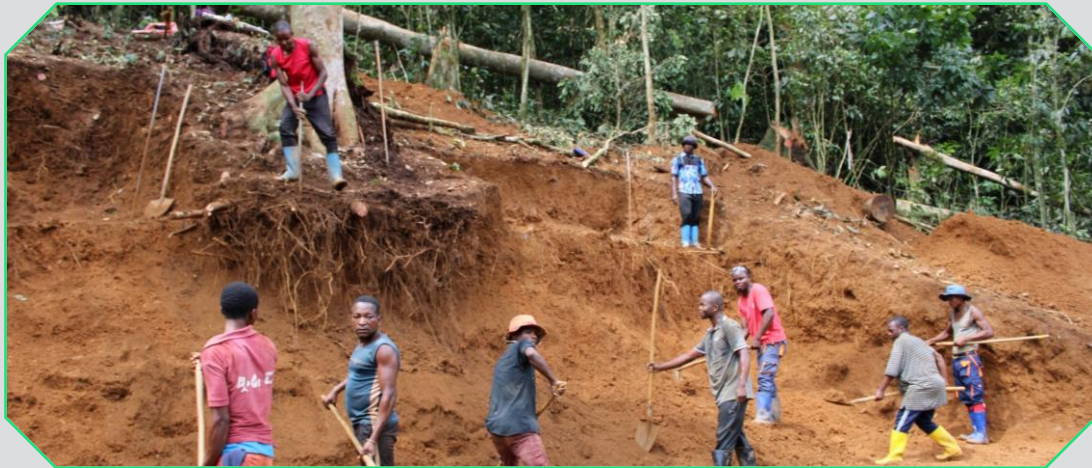
Drill core (cassiterite vein) and drill pad preparation
